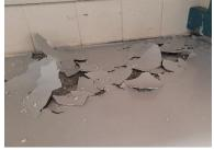
Injury and facility damage can occur from liquid nitrogen spills or from using inappropriate storage containers, like Styrofoam coolers, which are too porous to hold liquid nitrogen.
