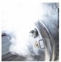
autoclave Adjusting inappropriately can result in uncontrolled release steam during cycle and building evacuation.
